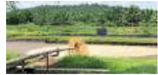
Figure 1: Palm oil mill effluent mixing pond.
